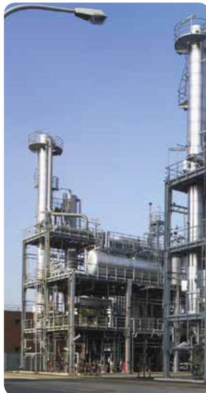
Chemical Processing Plants
