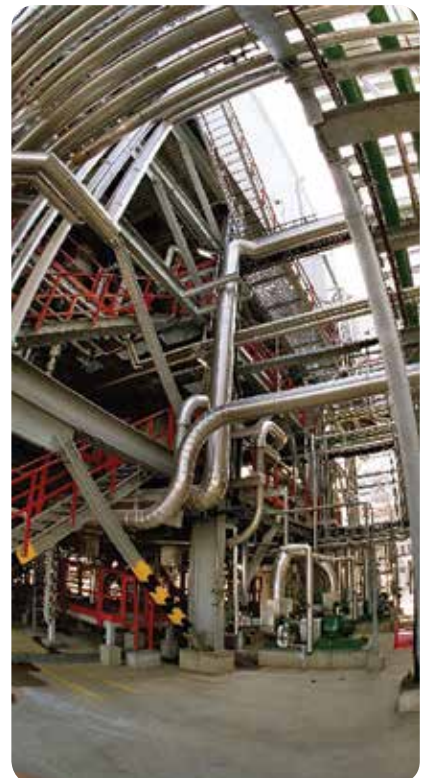
Metal Structure Coatings
