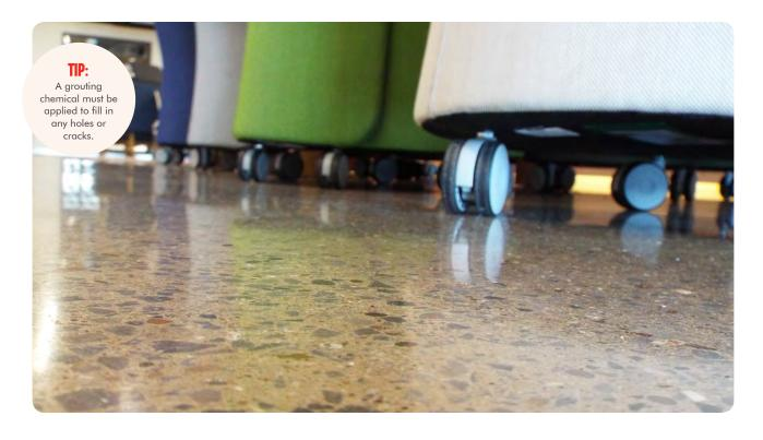
Polished concrete floors are susceptible to moisture and need to be properly sealed on both the top and the bottom. If liquid does manage to infiltrate the pores of the concrete then it could cause mould and mildew to grow, and if the liquid freezes it could lead to serious cracking in the slab.
