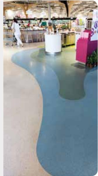
Complicated geometric or banded designs can be set out using aluminium or brass trims and the resin material poured into the design framework – similar to painting by numbers. Once ground, sealed and polished the stunning design reveals itself on the surface of the floor. This process can also be used to embed corporate logos or signage into the surface of the floor, which is often a unique touch in corporate offices or hotel lobbies.
